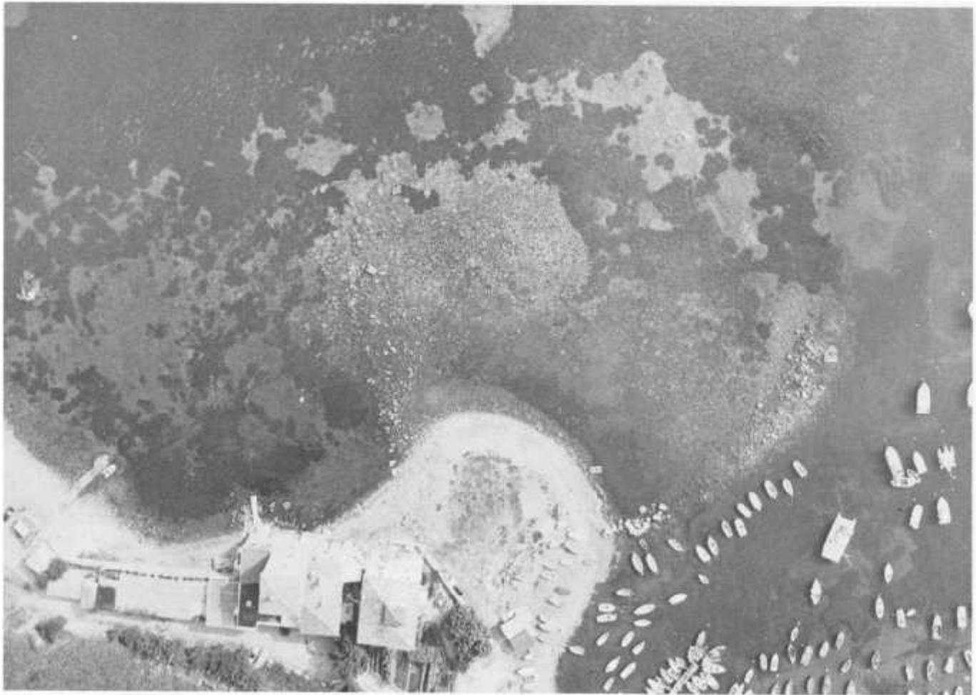
Figure 2. Aerial view of breakwater at Populonia. N is at top. Photo: J. Whittlesey.
