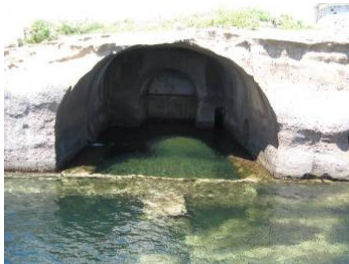
Fig. 14. One of the two covered pool of the Roman piscina complex. The water level, in the first century A.D., was ca. 1 m lower than at present. The wharf used for walking around the pool was then emerged, the tunnels visible in the picture dry. The niche for a statue is visible at the end of the room (Ph: A. Atauz).
